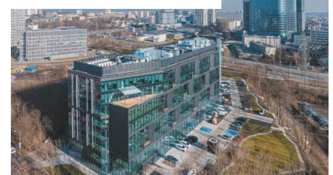
GRUNDMANNA OFFICE PARK, KATOWICE
