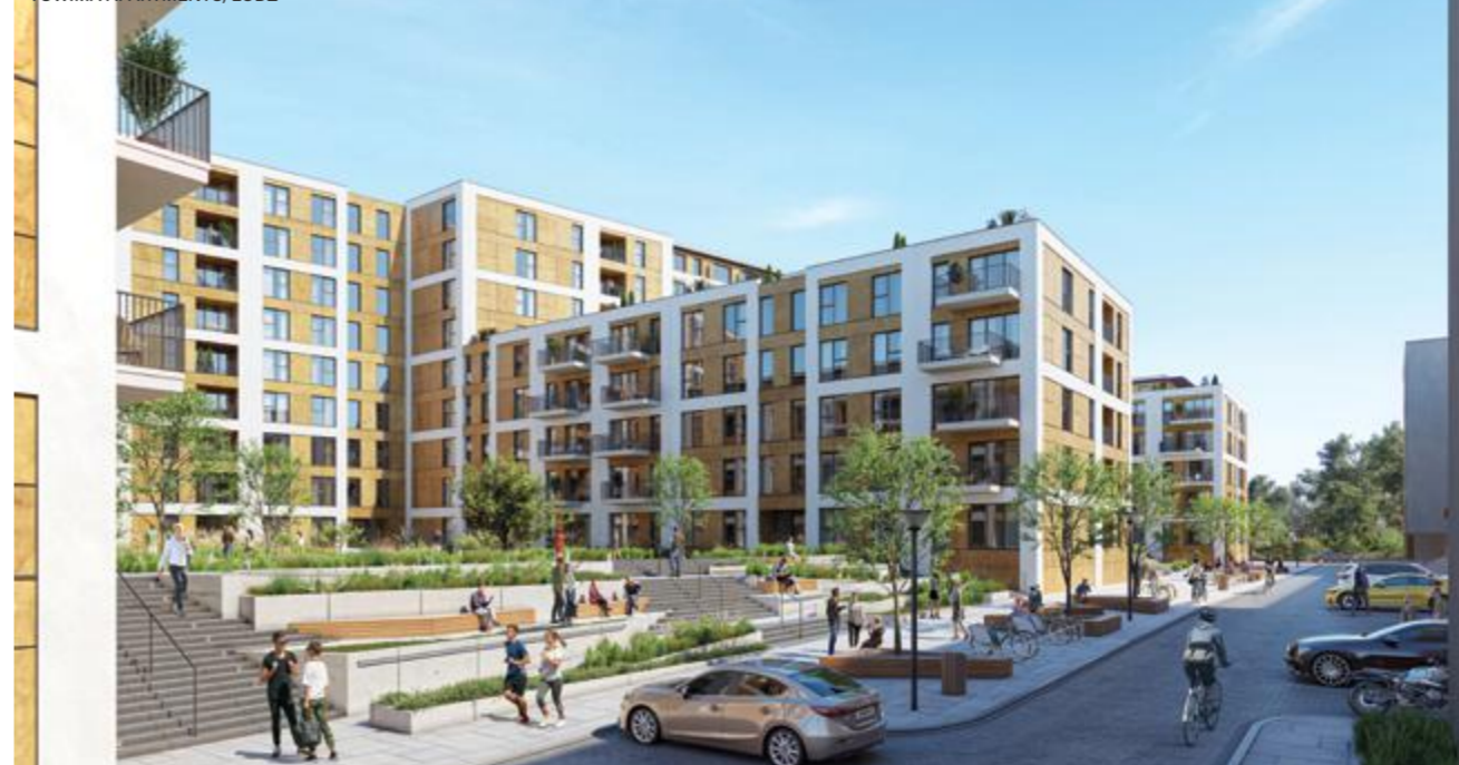
UWIMA APARTMENTS, ŁÓDŹ
